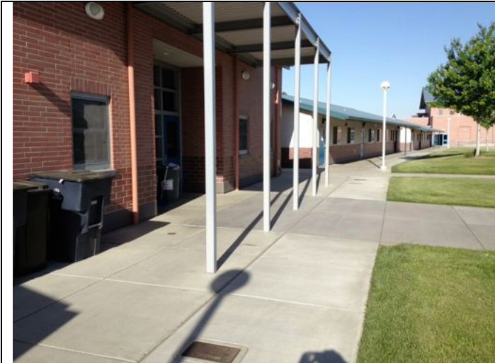
Expanded sidewalks and drainage improvements
