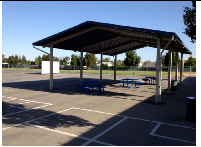
Shade structure in upper play yard
