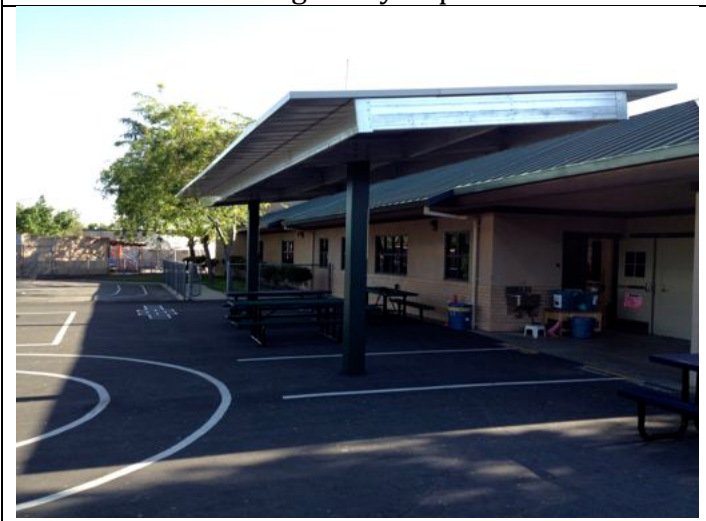
Kindergarten shade structure
