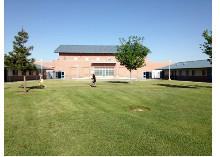
Removal of Hill and expansion of outdoor seating
