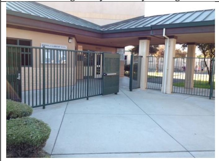
School fencing safety improvements
