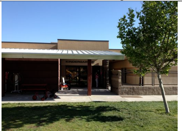
Kindergarten Shade Structure
